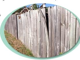
might be the result of rotting fence poles or loose bracing caused by our shifting soil. Consider switching to metal poles and resetting your concrete.
